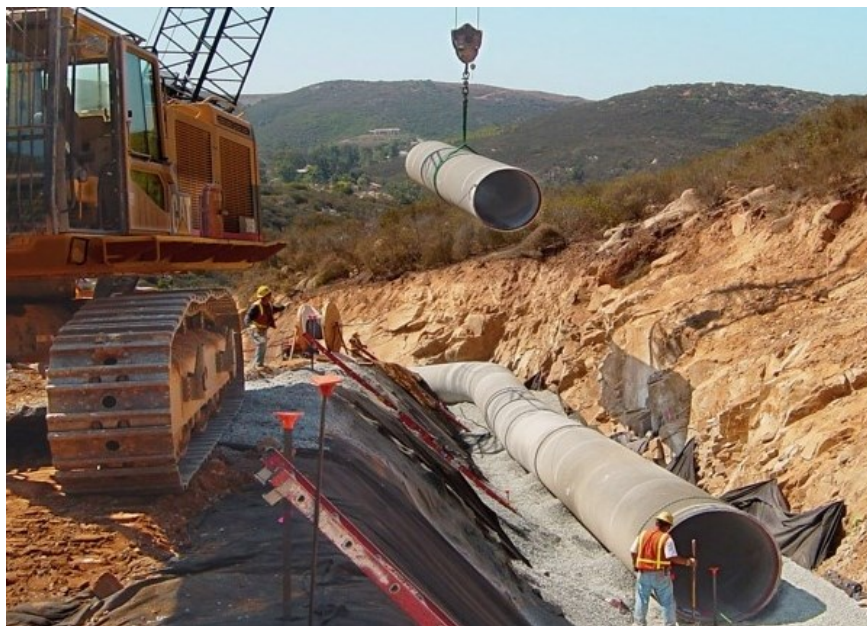
Construction of water transmission pipelines. © SDCWA
